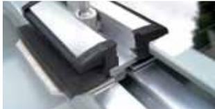
Example of a one-part clamp with underlayment plate
