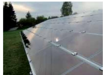
Horizontal mounting of laminated (thin-film) modules
